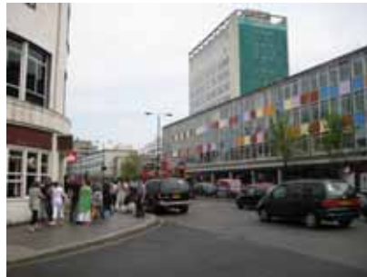
A proposed major refurbishment of the 1960s buildings?
