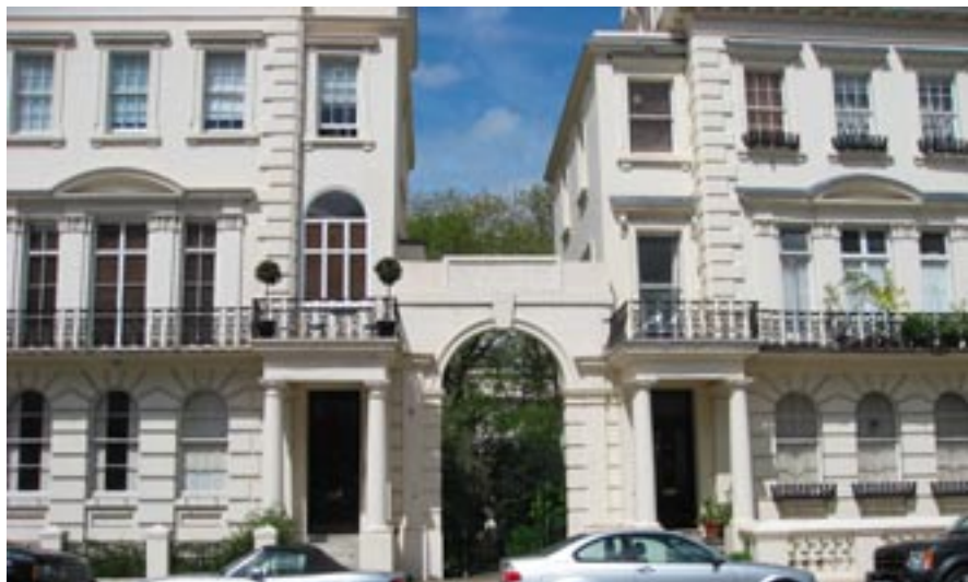
Ornamental arch in the gap between 33 & 34 Kensington Park Gardens, in the middle of the terrace.
