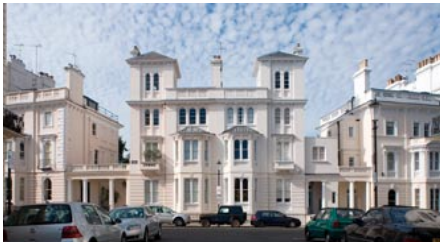
Porticos in the gaps between houses in Stanley Crescent, one portico untouched, the other with subsequent extensions. ©Thomas Erskine
