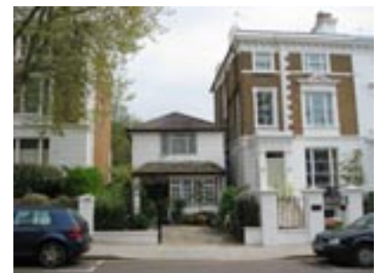
The house in the gap between 22 & 24 Lansdowne Road.
