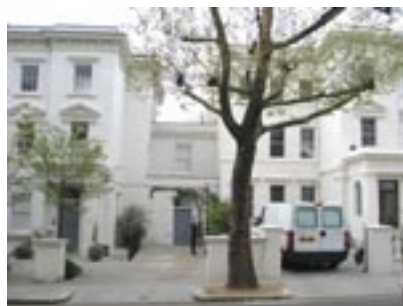
Uncoordinated infilling between Nos. 39 & 40 Lansdowne Road.
