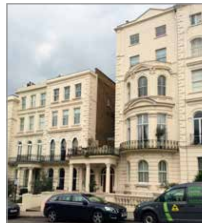
64, 66 and 68 Ladbroke Grove
