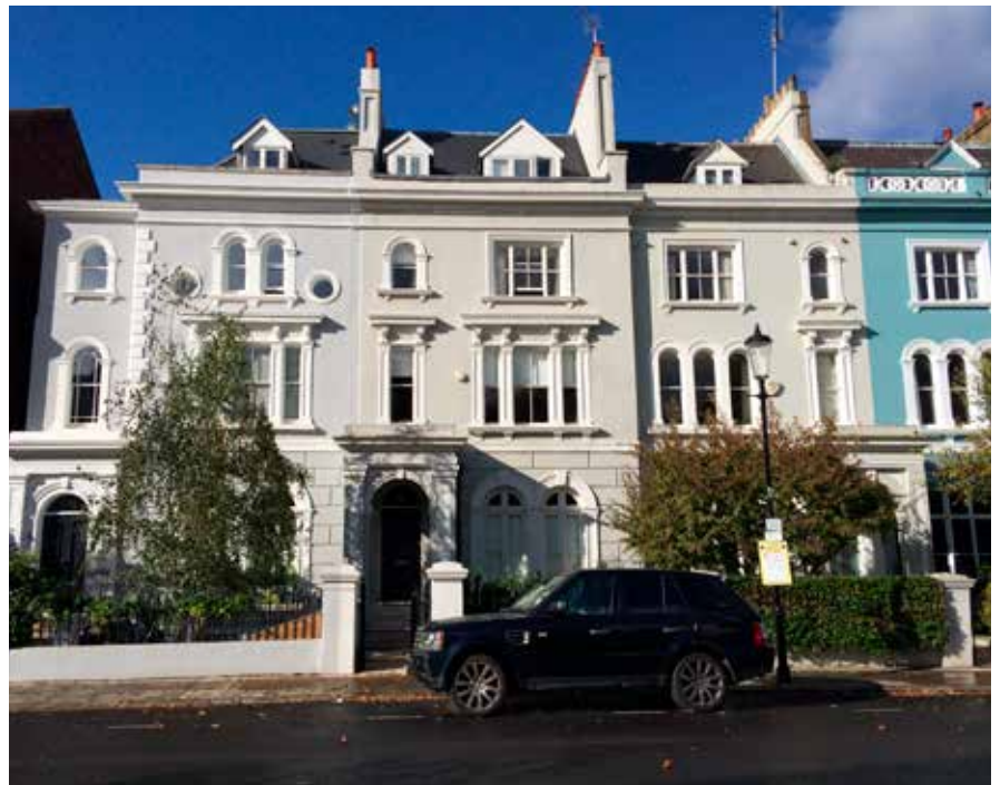
End of terrace in Elgin Crescent. The two end house are set slightly forward of and have different windows from the mid-terrace houses. This is replicated at the other end of the terrace.
